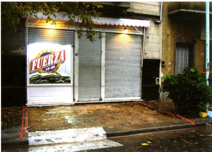
General view of the gallery's façade after repairs.
